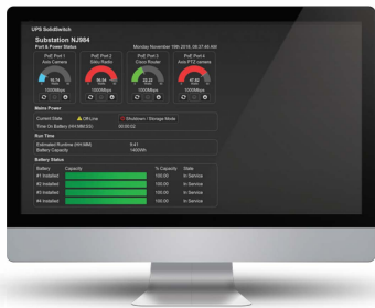
UPS-SolidSwitch Command Post
